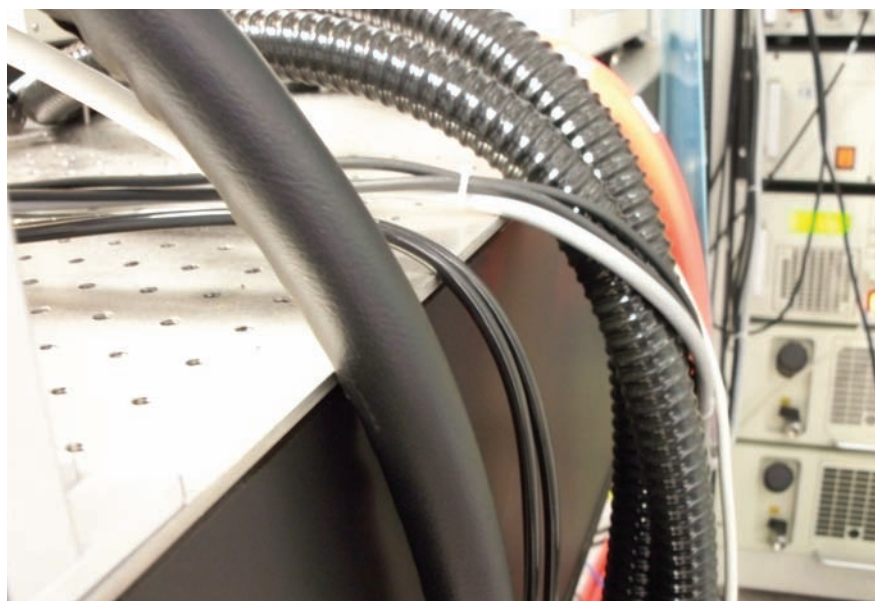
Figure 5. Tight hoses hanging off platforms like those shown can transmit vibrations directly onto the table surface. These cables should have some type of foam isolator placed under them or be supported so they do not touch the table.
