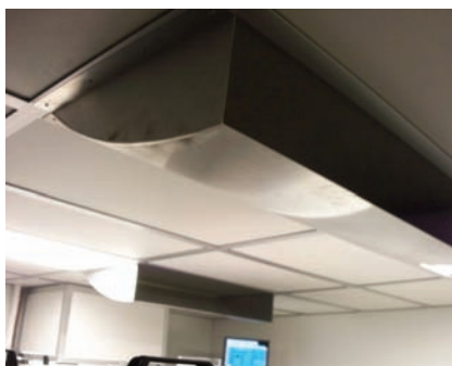
Figure 7. Air duct baffles redirect airflow and will help reduce tabletop disturbances while maintaining proper lab temperatures.
